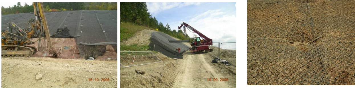
Figure 12...14: construction moments in a slope of mudstone; in figure 12..13 the surface starts to cover with the erosion protection mat
