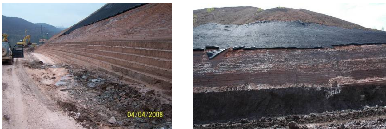
Figure 19...20: Erosion protection on a potash tailings pile (during construction)
