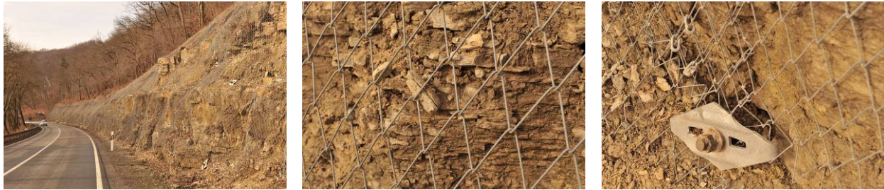
Figure 16...18. A bad example: Details of slope retaining in Muschelkalk WITHOUT erosion protection 6 months after completion
